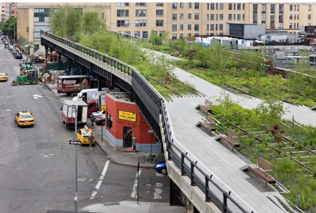
High Line, 2009. Manhattan, Nova York James Corner Field Operations
